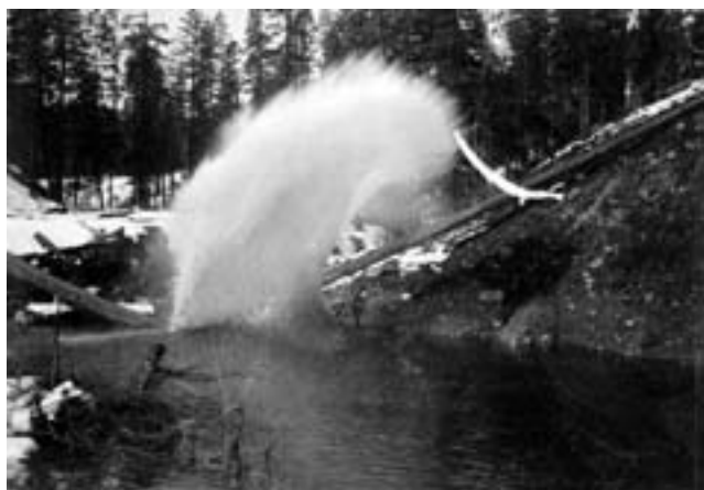
Log chute coming down slope at right. Flumes used water to float the logs on their trip; chutes used gravity (and sometimes grease). Photographer: Eastman.
