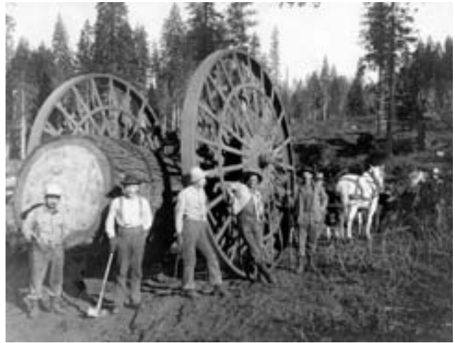
“High Wheels” sometimes called “Big Wheels.” This type of equipment was used by Brooks-Scanlon Lumber Co. and other companies until replaced by tractor logging (later called Cat logging because of the company that made many of the machines). Photographer: Miller, 1903.
