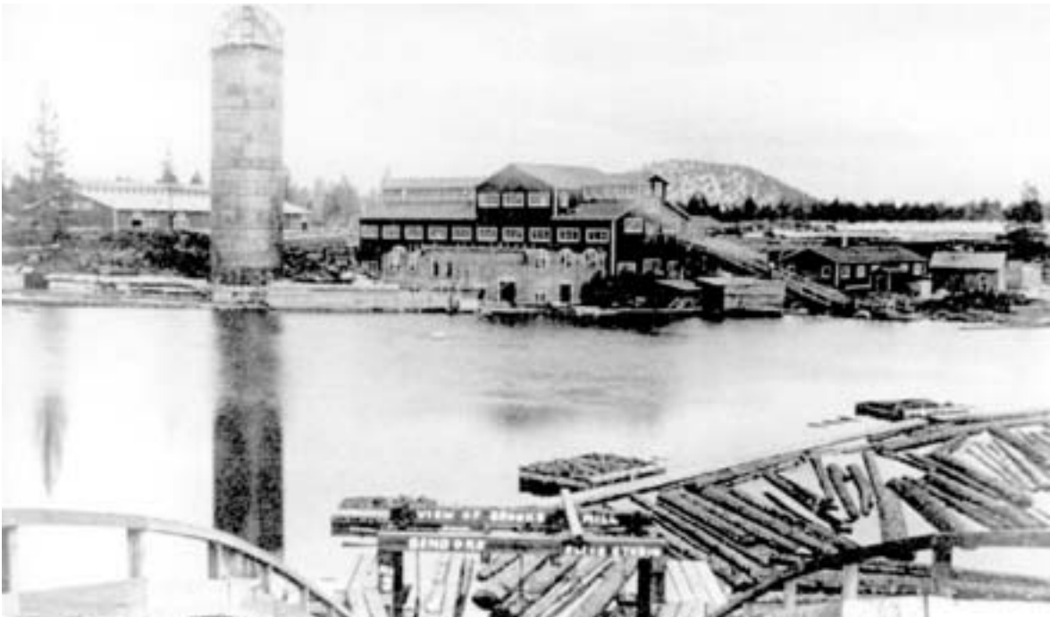
Mill at Bend after reconstruction, about 1917.
