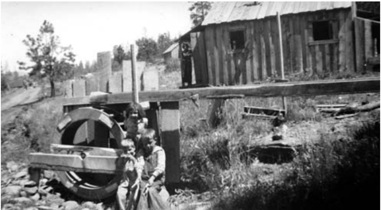
This is the water wheel power source that Duke Dotson built for his family. The Dotsons were the only family in the camp to have electricity. This is on Fort Creek on the south edge of the camp.
