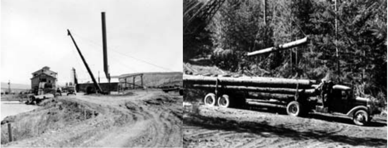
Left, log dump at an early date before plant is completed. Right, loading logs in Ochoco's timber. Unless otherwise noted, all photographs are from the Kelly collection, graciously loaned to me by Paul's daughter, Jean Zell of Portland.
