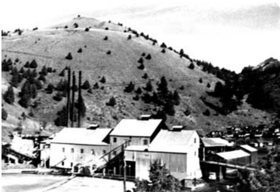
Main mill building with the camp in background. Three stacks are from power house. Ellingson had dry kilns at Izee (out of sight behind the main building). Mill scraps were taken by conveyor from mill building to the wigwam burner across (north) the river.
