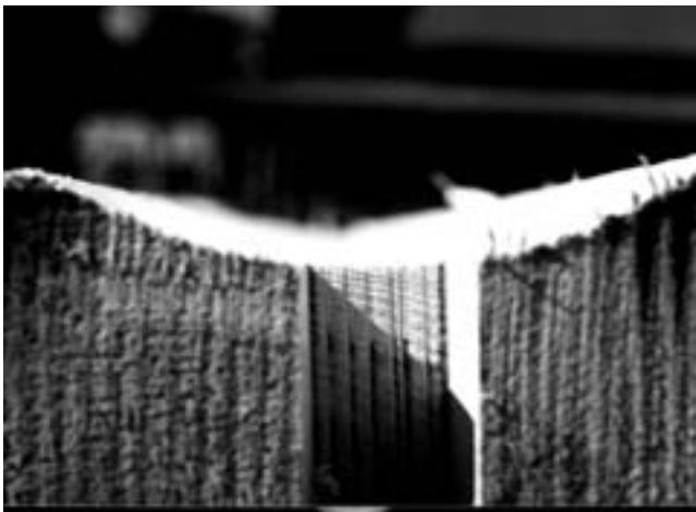
The concave cut and vertical groove, both of which receive insulation strips between adjoining logs.
